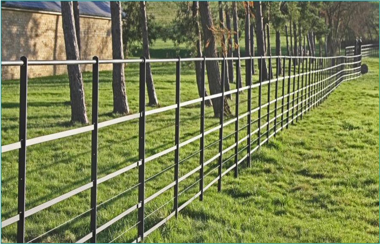
Fig. D12 - An example of estate railings.
