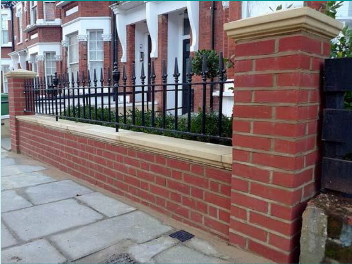
Fig. D10 - An example of a dwarf wall with railings.
